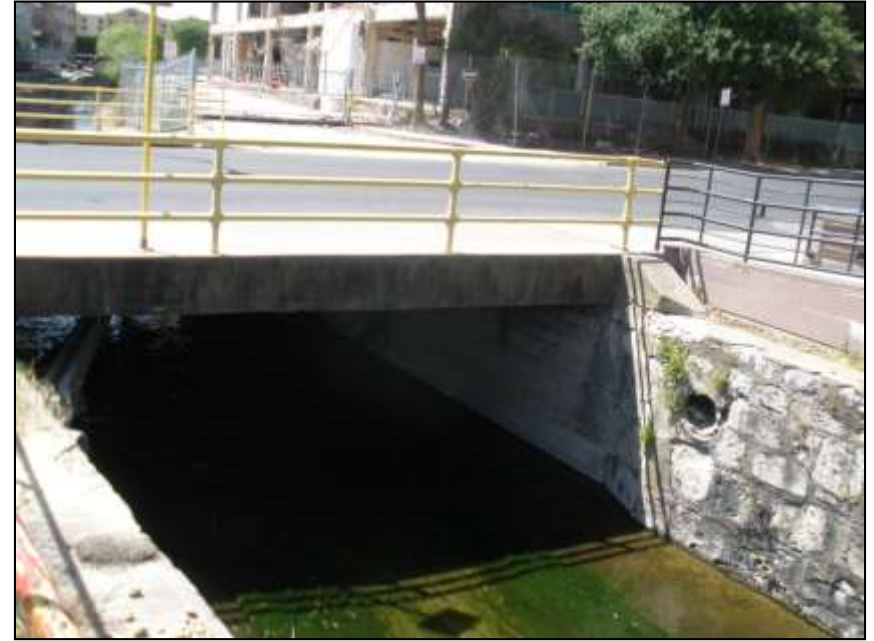
Vehicular bridge at W. Nueva
